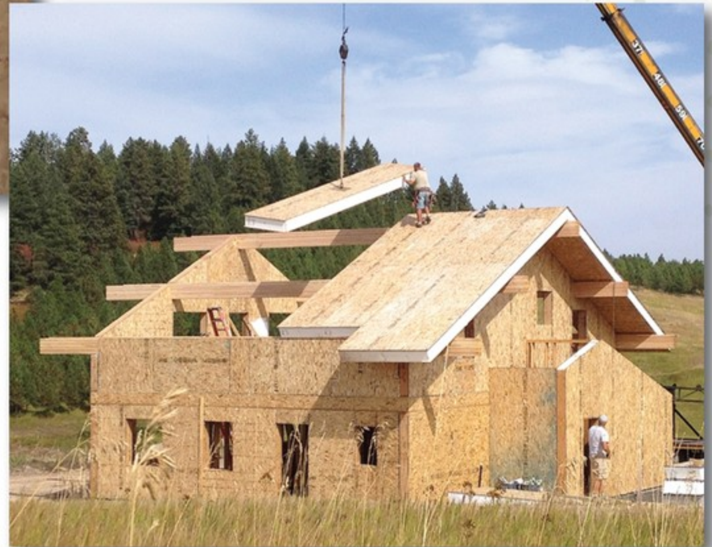
▲ Compared to traditional stick-frame construction, assembly of the panels on-site saves enough time and labor to make SIP a competitive cost-effective solution.
