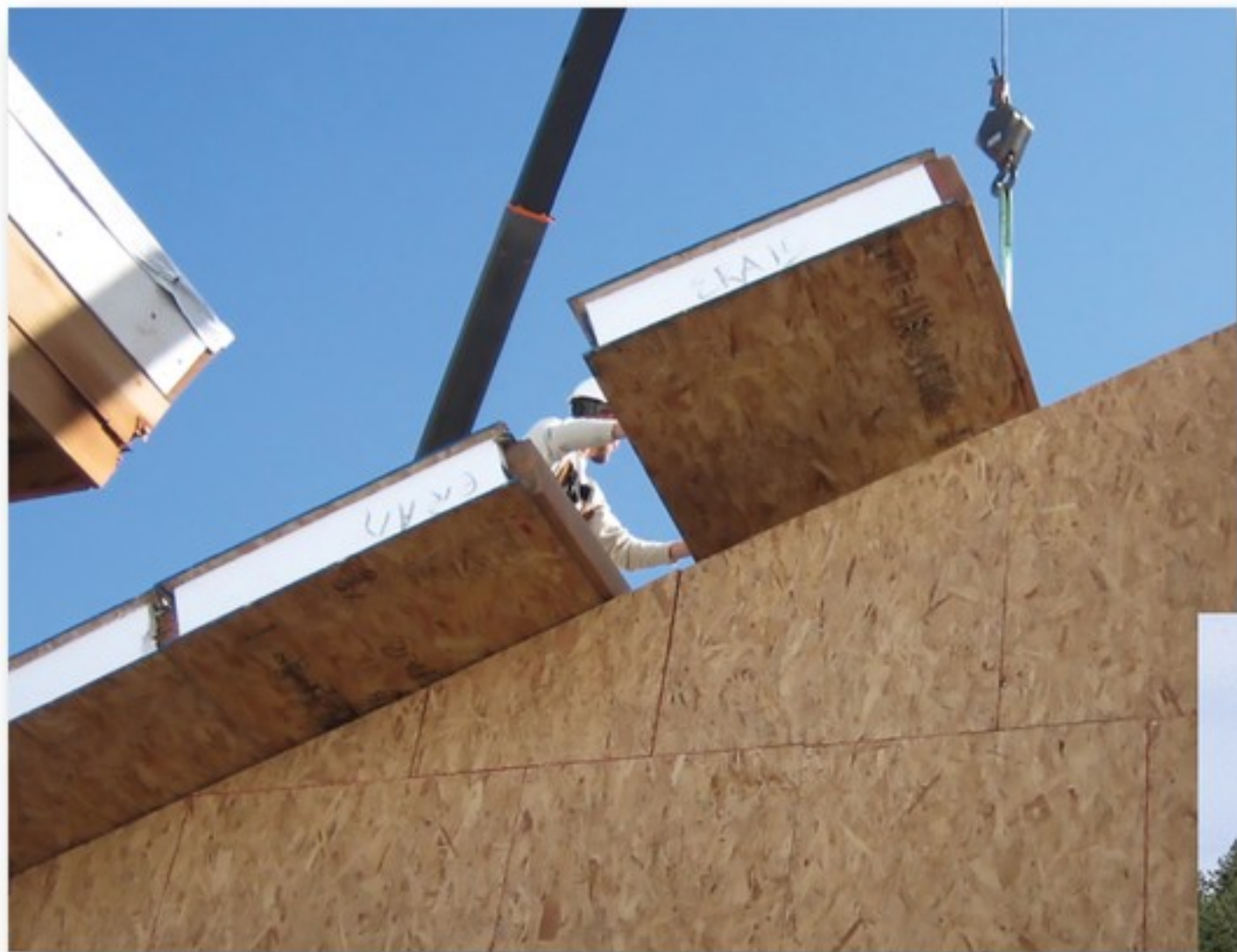
▲ Close-up of the 12-inch SIP roof panel being hoisted into place.
